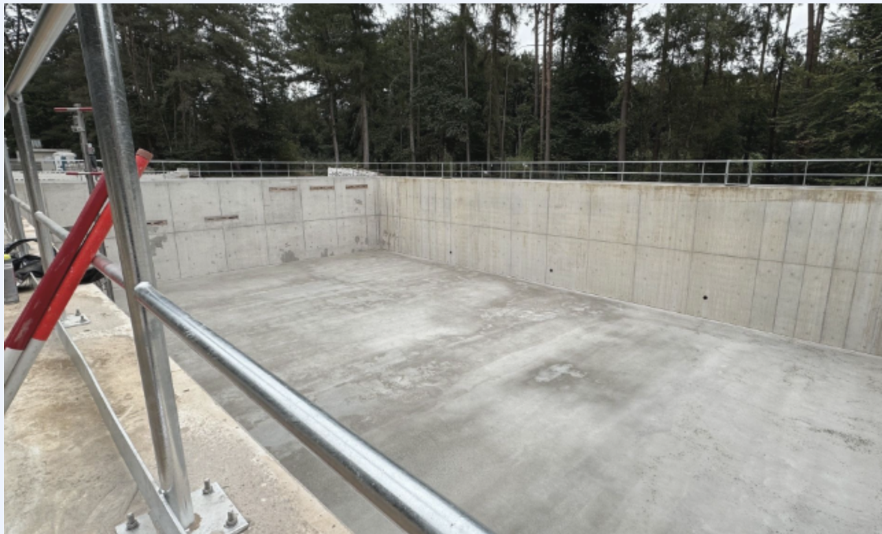
Das fast fertige Becken in Braschoß (Foto: SBS)
